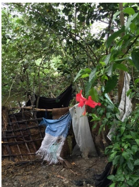
Figure 2.18: Typical Hanging Latrine used widely by respondents in earlier phases of CDSP (picture from South Hatiya Polder, the canal is just visible though the undergrowth)
