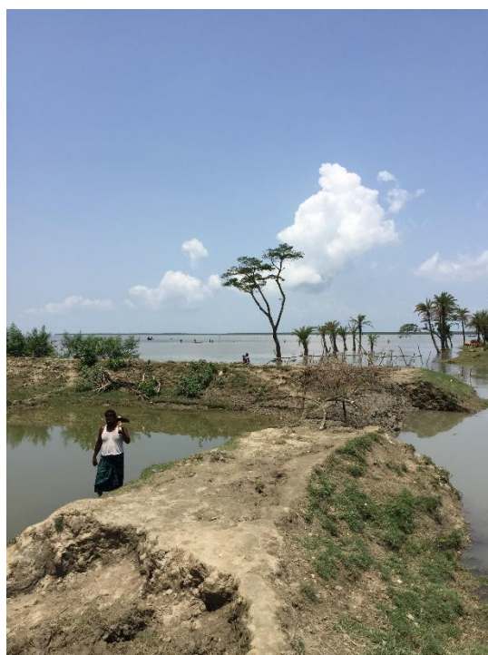
Figure 0.4: State of Erosion of Secondary Embankment along west coast of Hatiya, Tamaruddin Union
